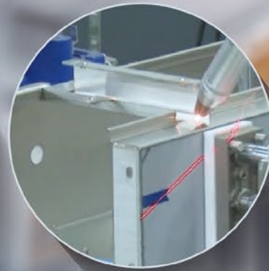
Automatic Laser Welding
